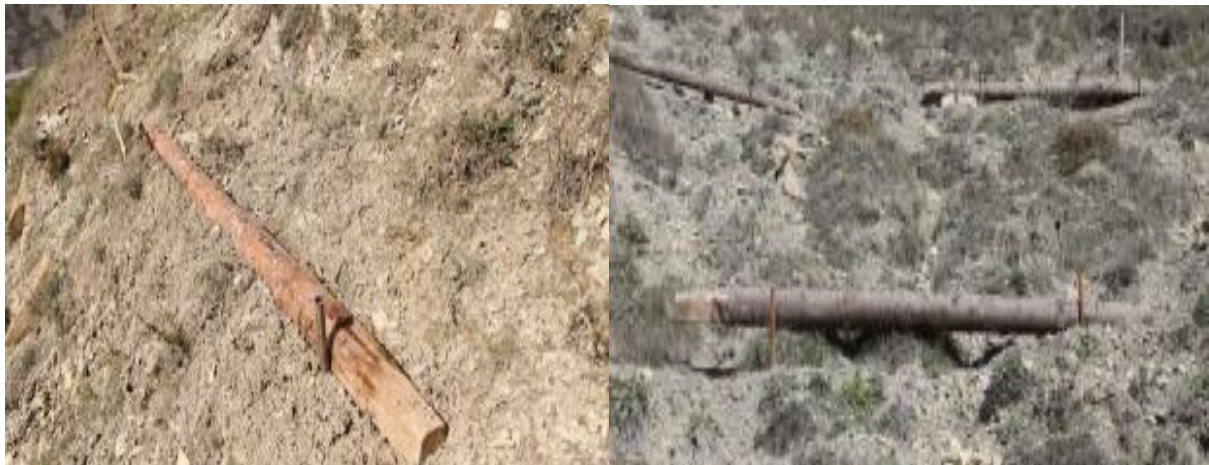
Figure 9: The height of the timbers is low and bottom line of the pile walls is empty
