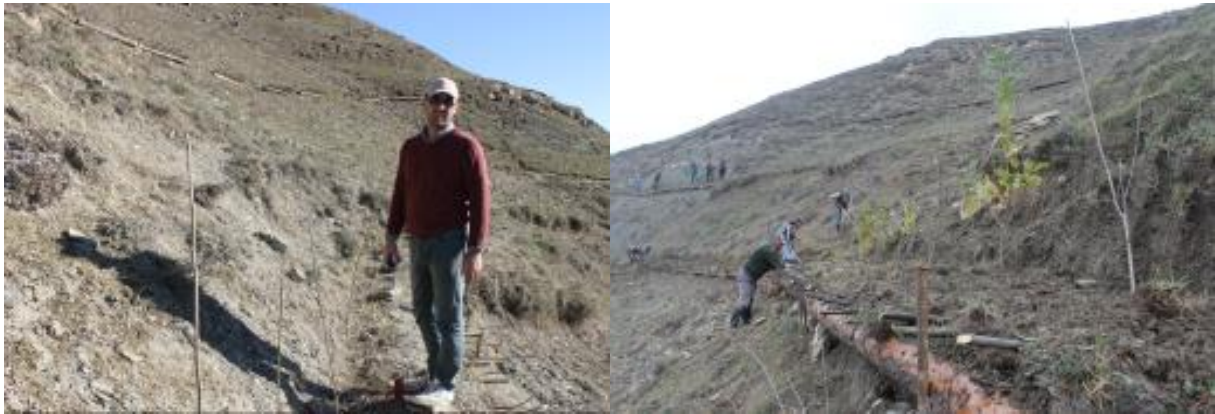
Figure 18: Tree planting and live stakes of willow on the pile walls
