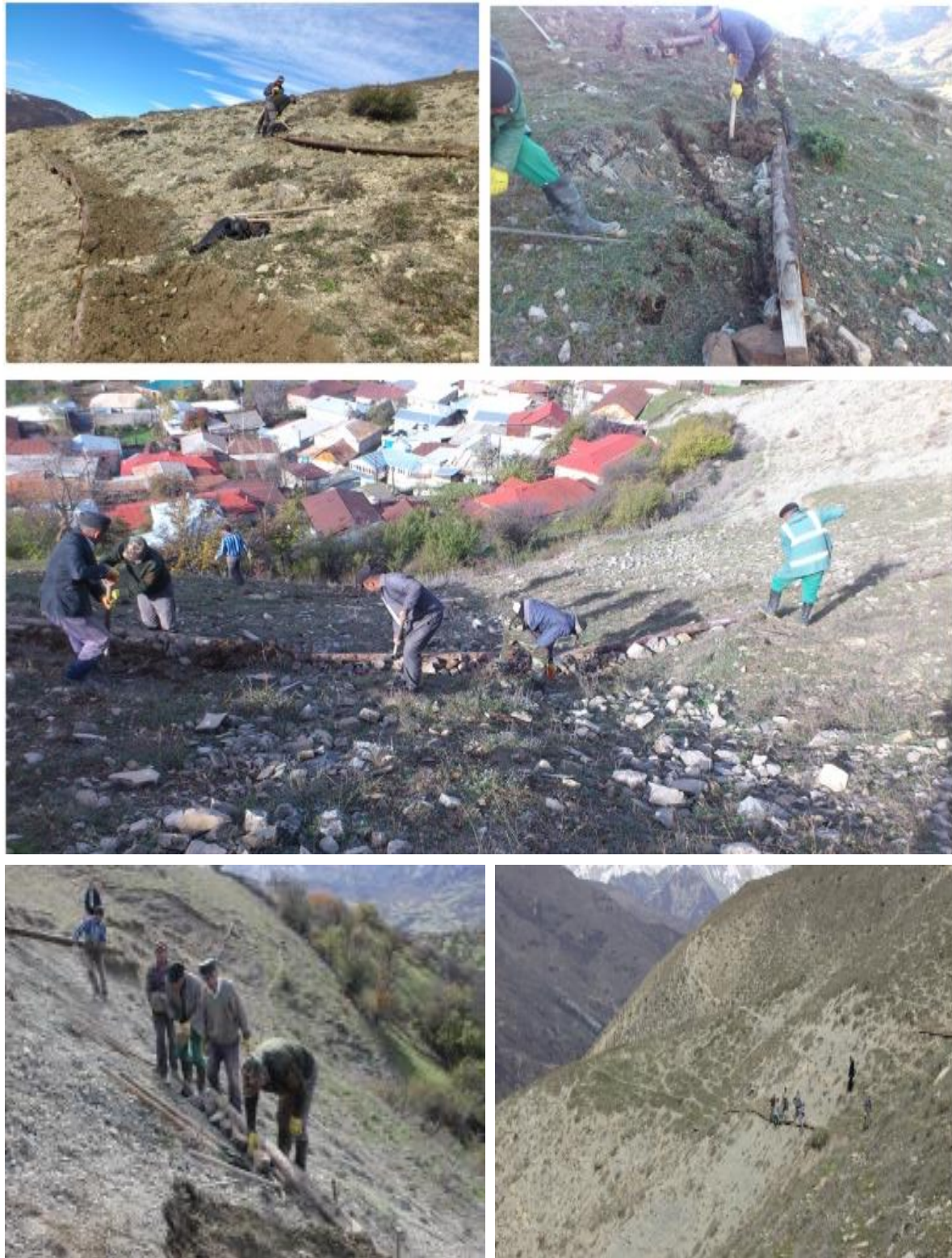
Figure 11: The timbers are raised and the positions of the pile walls are changed
