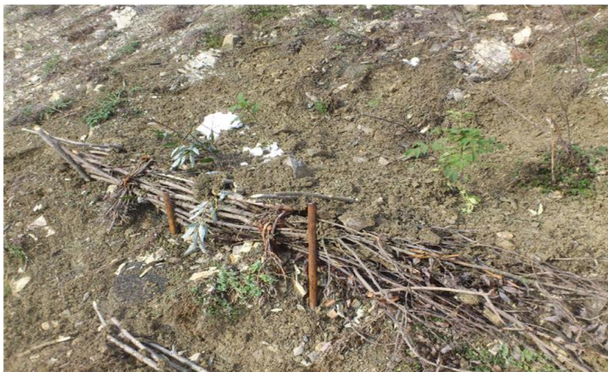
Figure 14: The bunches of long twigs can be used in constructing pile walls
