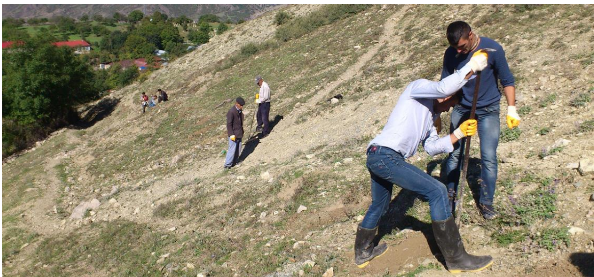
Figure 6: In rocky ground community members used traditional metal crowbars to dig holes
