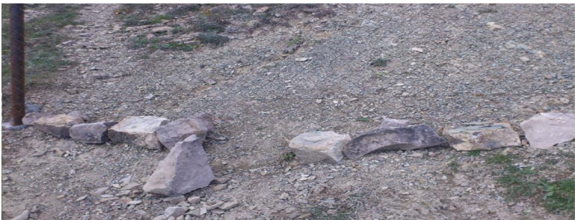
Figure 8: The bottom line of the permanent wire net needs to be closed
