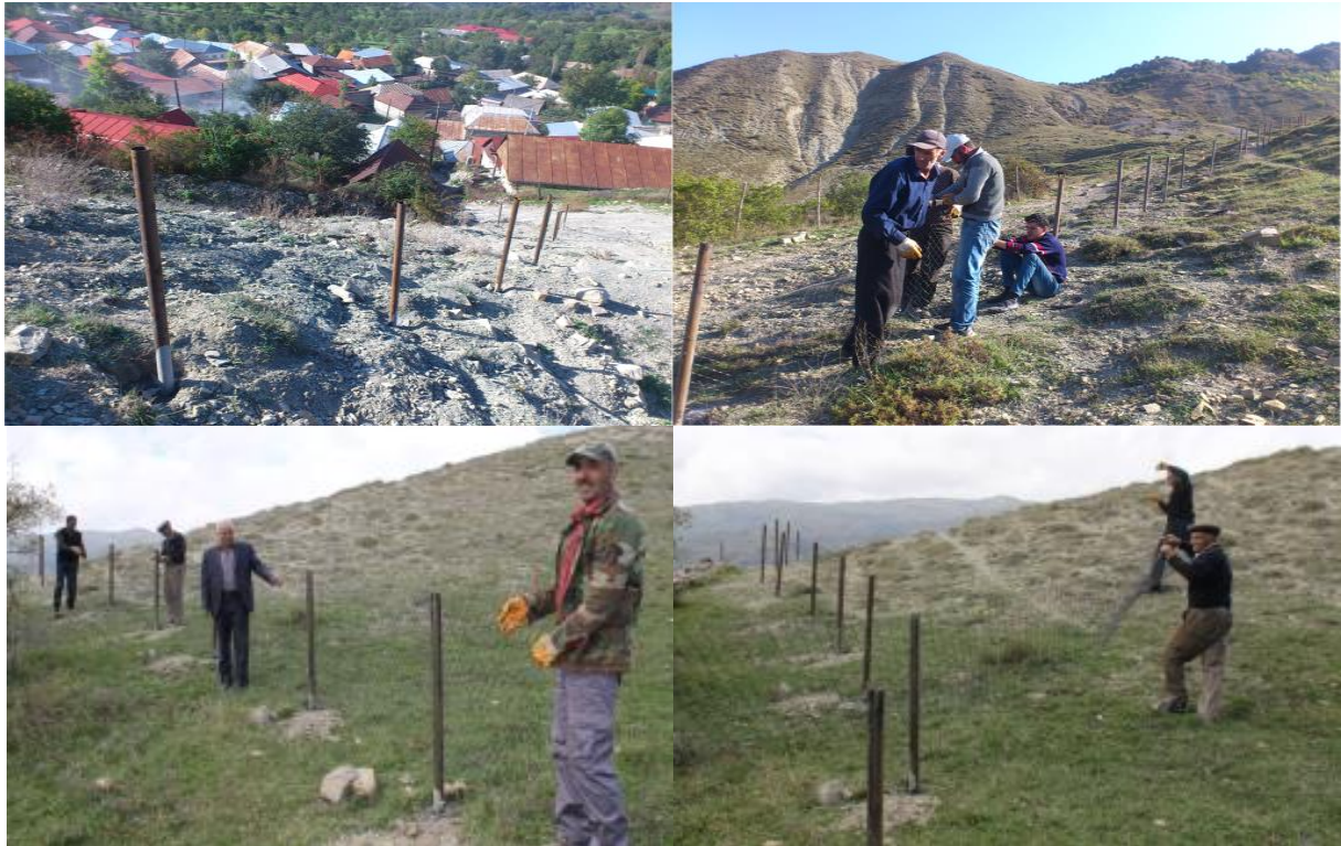
Figure 7: Poles were fixed with concrete and fence is installing
