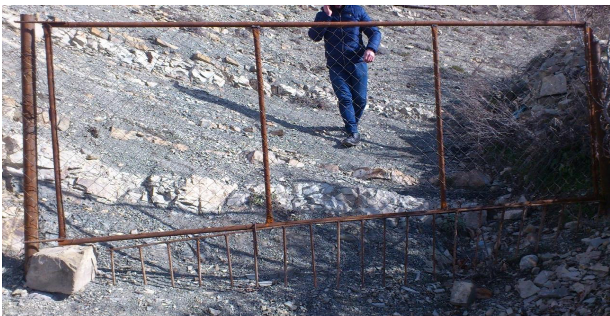
Figure 13: The bottom line (open entrance) of the gate was closed with a movable extension
