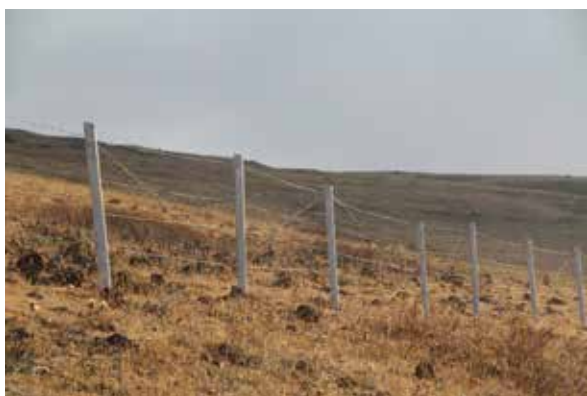
Fig.2: Installed barb wire fence at the upper plot in Nahapetavan
