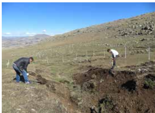
Fig. 3: Flattening of gully shoulders
