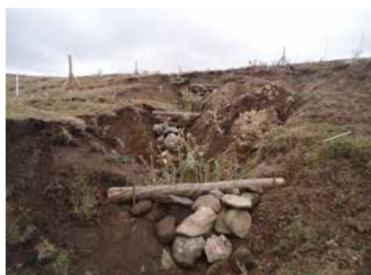
Fig. 6: Fortification of check dams with rocks and stones
