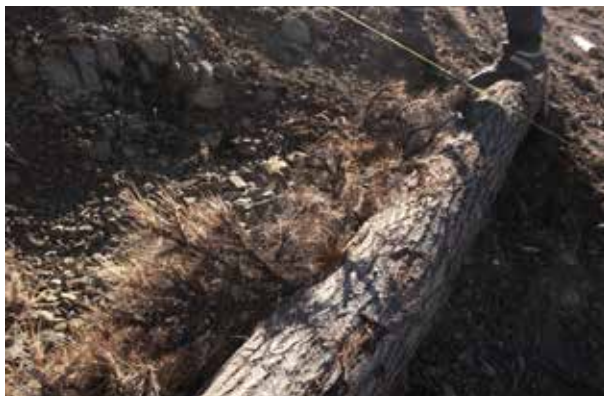
Fig. 4: Filling up the area behind the wooden log with soil and plant material (left) and covering open soil with hay (right). November 2016
