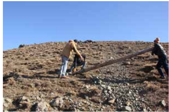
Fig. 3: Putting logs in correct position across the slope (November 2016)
