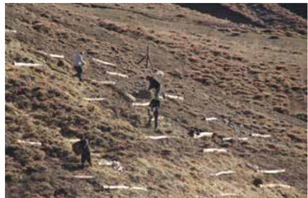
Fig. 4: Filling up the area behind the wooden log with soil and plant material (left) and covering open soil with hay (right). November 2016
