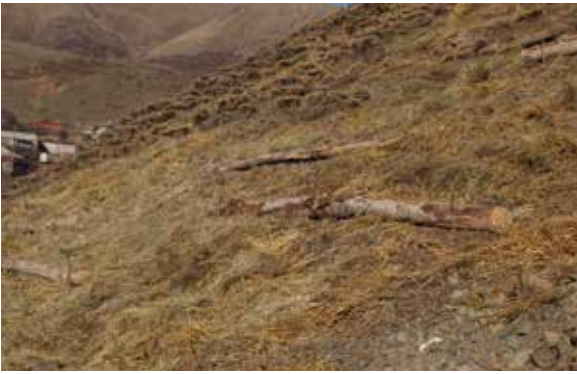
Fig. 5: Pile walls and mulching are applied to combat advanced sheet erosion on a slope
