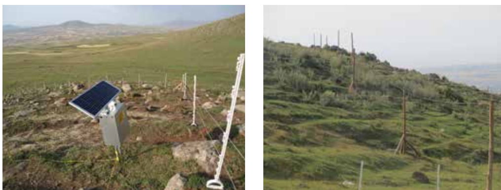
Fig. 2: Electric fence with solar panel (left) and above ground connection (right)
