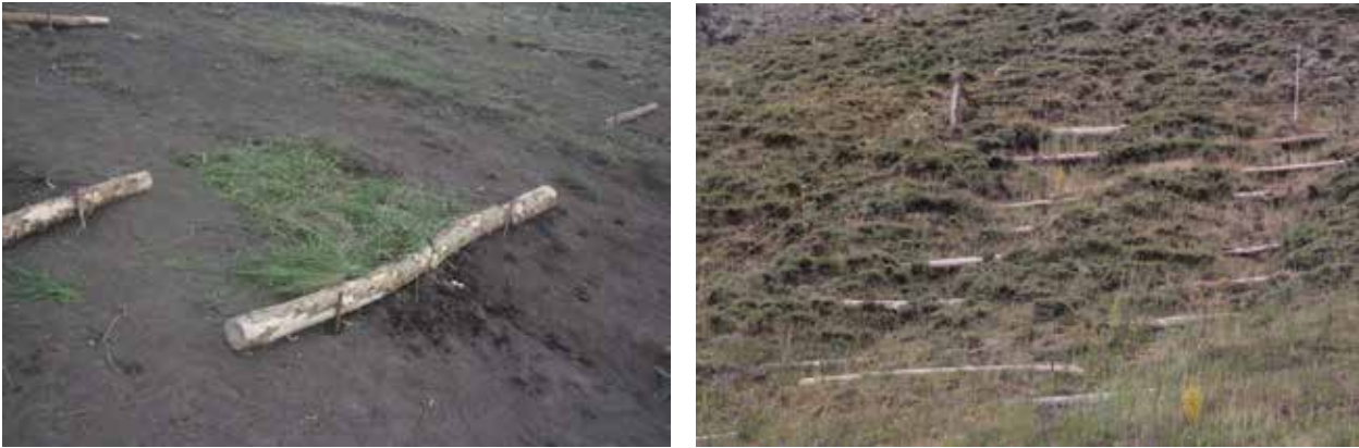
Fig. 5: Examples of pile walls on different pilot sites. Offset establishment of pile walls (left) and below each other in water run-off grooves (right)
