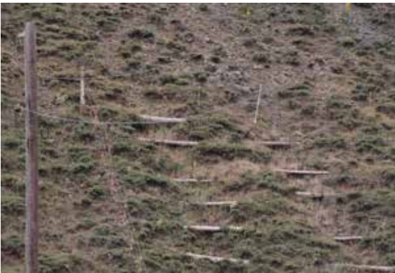
Fig. 6: Pile walls to combat rill erosion
